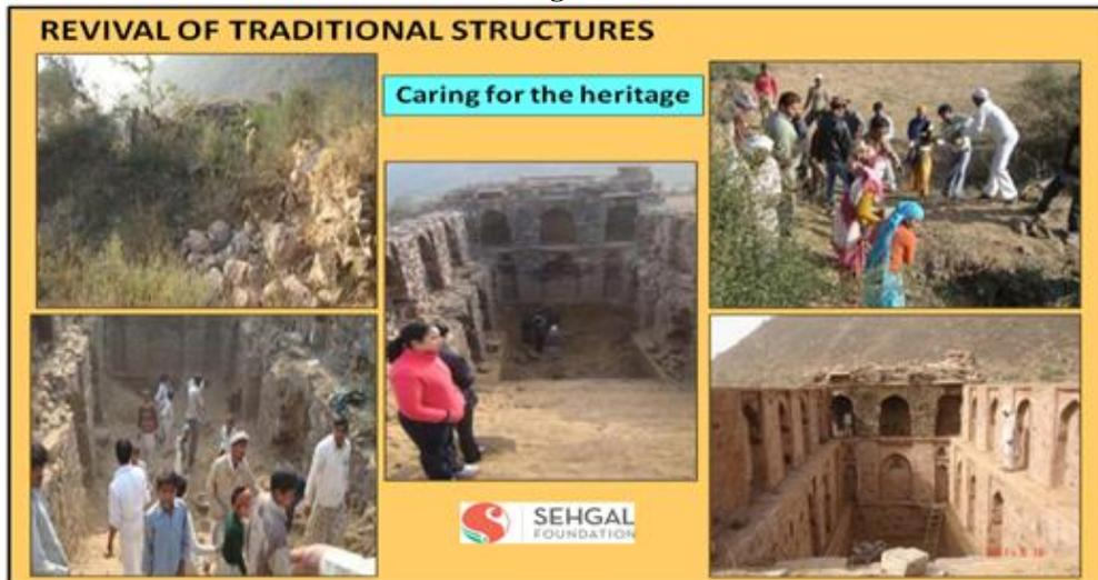
The structure shown in the photo (left) is a 500-years-old stepped well, which had lost its capacity to catch and hold monsoon runoff and store it for dry seasons. After revival, the structure helps in recharging groundwater using rains.
