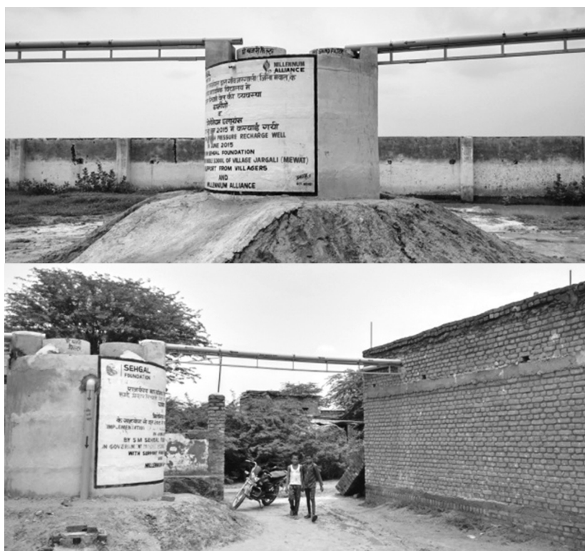
The cylindrical tank built over the ground to collect the water from the high-pressure recharge well, Government High School, Sukhpuri, Nagina block
