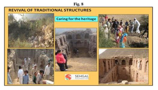
The structure shown in the photo (left) is a 500-years-old stepped well, which had lost its capacity to catch and hold monsoon runoff and store it for dry seasons. After revival, the structure helps in recharging groundwater using rains.
