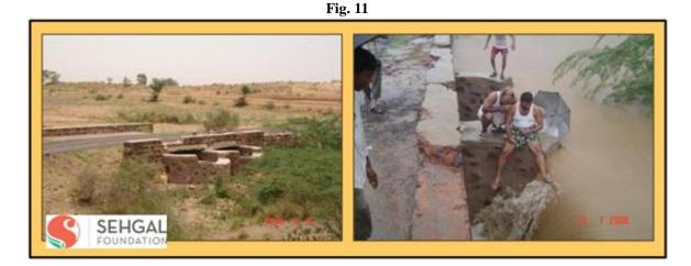
The concentration of runoff is reduced on downstream, helping in preventing loss of fertile soil due to erosion by increased runoff pressure. Such a process is highly effective and needs minimal cost input. Culverts can:
