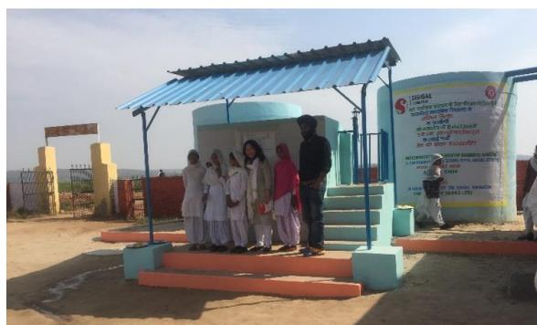
To address the issue of safe drinking water, a component of Sehgal Foundation's Transform Lives *one school at a time* initiative builds rainwater harvesting (RWH) systems with biosand filtration that provide safe drinking water to schoolchildren. This system collects rainwater for storage in over or underground tanks that passes through a filter before being available for
